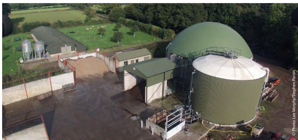
Figure 24: Small biogas plant on mixed sheep, dairy and free-range chicken farm
