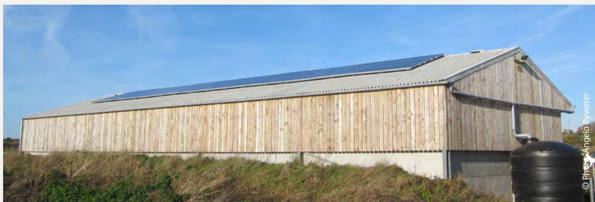
Figure 31: Solar PV and rainwater recovery
