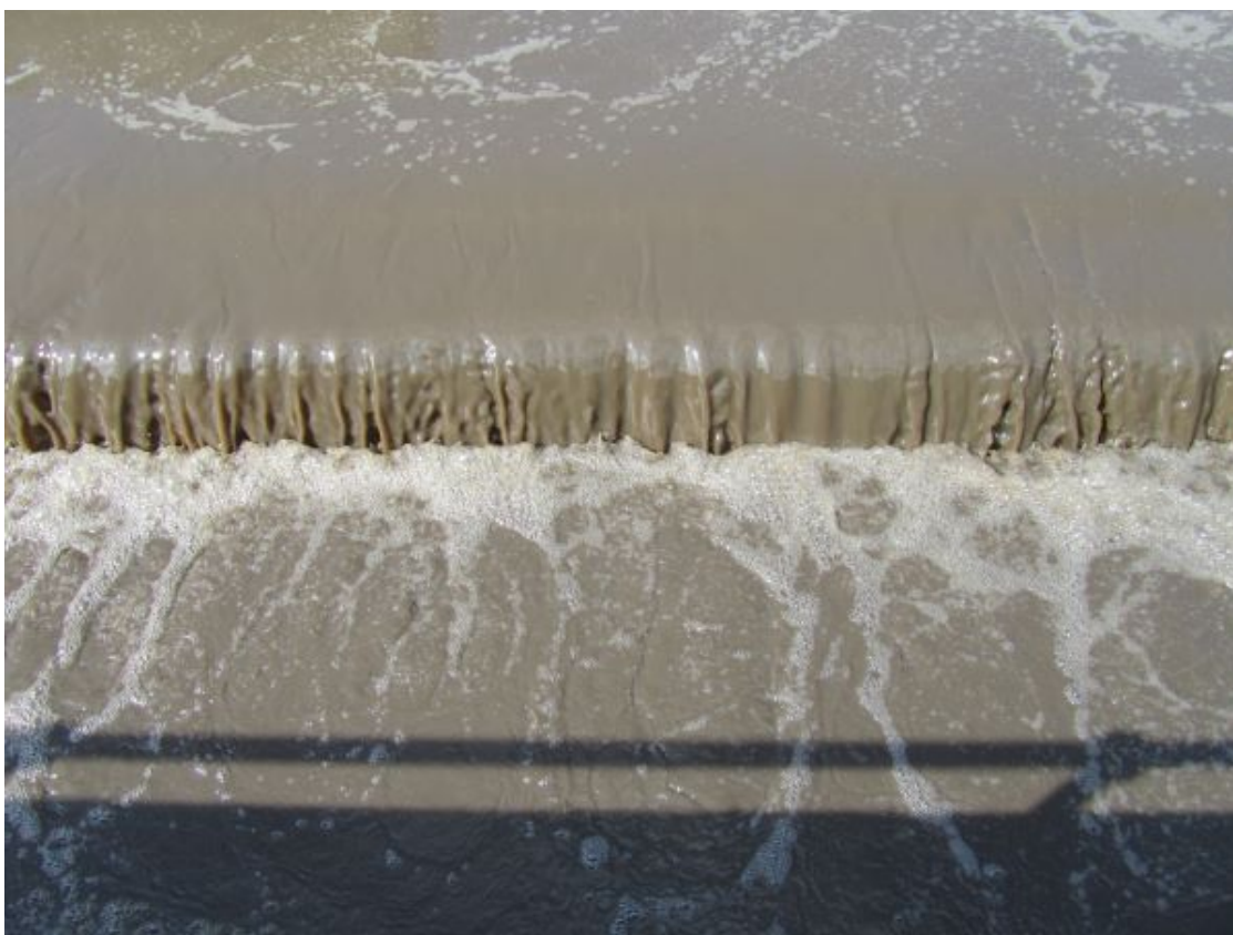
Image of weir in an Activated Sludge plant courtesy of Prof Charles Banks
